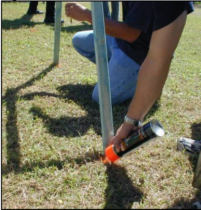
Marking the contour line with spray paint
