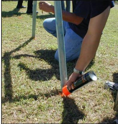
Marking the contour line with spray paint
