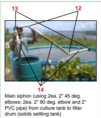
Main siphon (using 2ea. 2" 45 deg. elbows; 2ea. 2" 90 deg. elbow and 2" PVC pipe) from culture tank to filter drum (solids settling tank)
